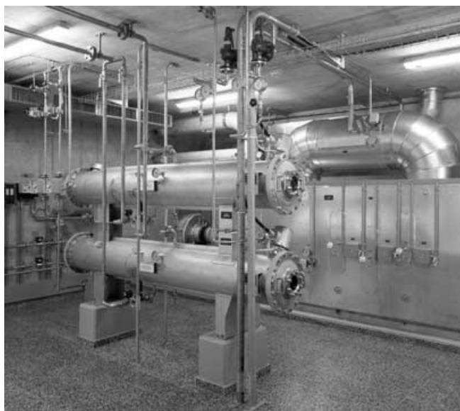
**Figure 14** | Ozone plant production 0.3 kg/h to 2.7 kg/h.
