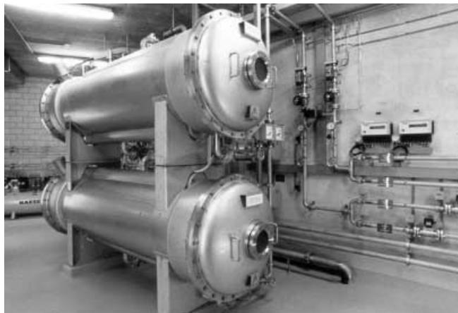
**Figure 13** | Ozone plant production 1.25 kg/h to 12.5 kg/h.
