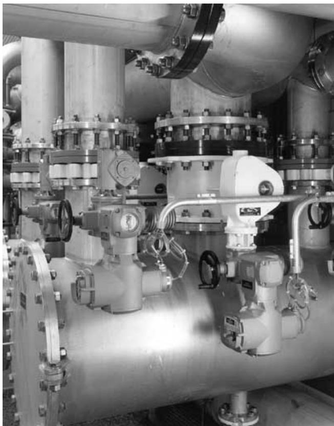
**Figure 12** | Buffer room entry with filtrate washwater and cleaning air inlet.
