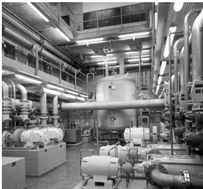
Figure 9 | Piping cellar Küssnacht/Erlenbach water lakewater treatment plant.
