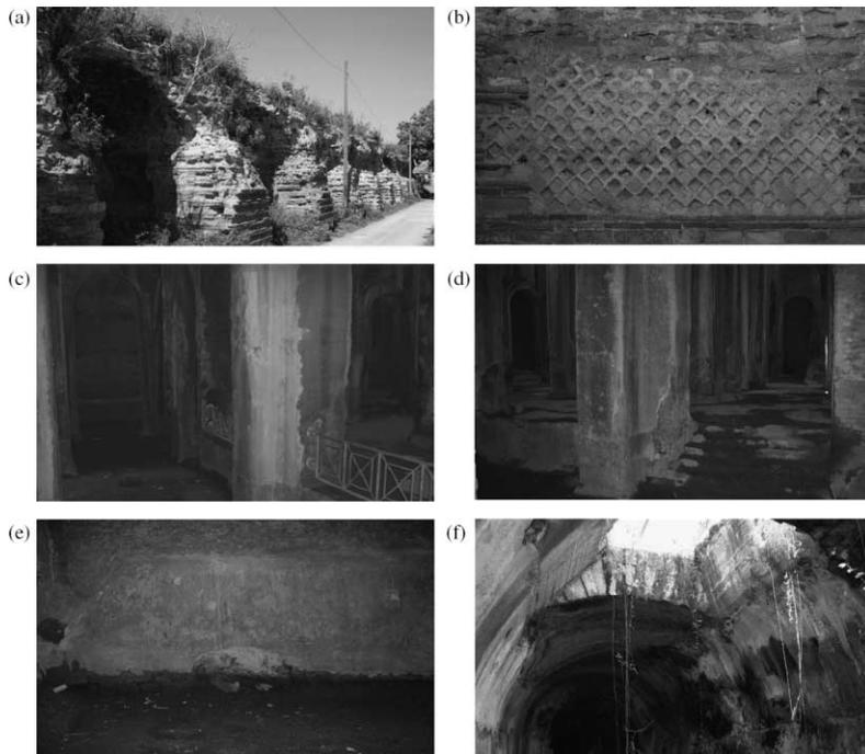
**Figure 4** | Images of the Piscina Mirabilis: (a) outside barrel vaults; (b) particular of *opus reticulatum* of the wall of an outside barrel vaulted niche; (c) internal *Piscina Limaria*; (d) one of the two *Piscina Limaria* staircase; (e) discharge hole in the *Piscina Limaria*; (f) a hole in the barrel vaulted roof.
