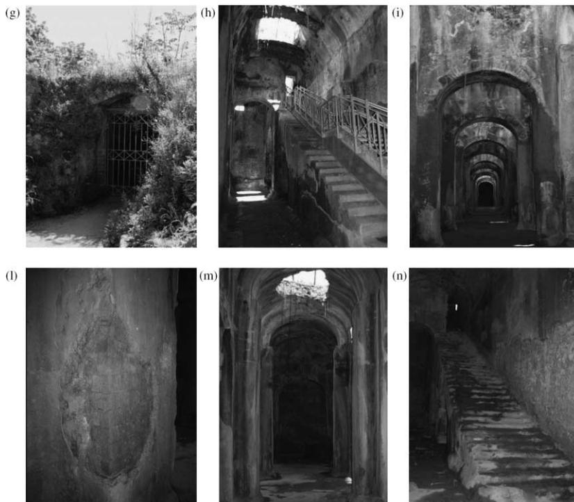
**Figure 5** | Images of the Piscina Mirabilis: (g) the northwest entrance near the inlet water; (h) the northwest staircase (inlet water); (i) a longitudinal aisle; (l) a tufa stone pillar covered with a thick waterproof layer of *opus signinum* (pounded terracotta); (m) a cross aisle; (n) the northwest staircase (the ancient Roman entrance).
