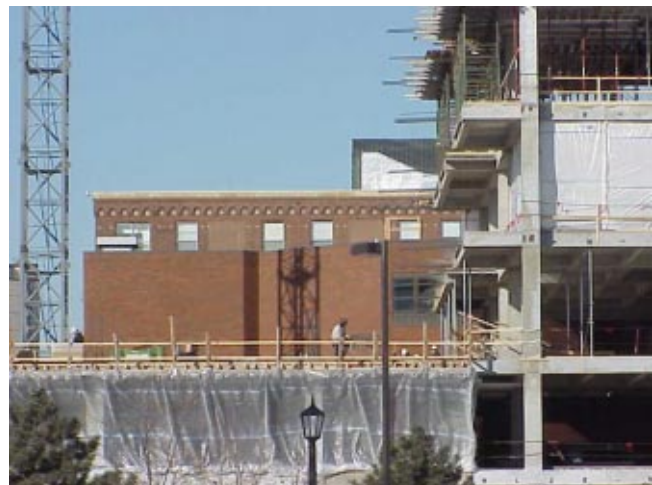
Fig. 1 Photograph of new construction in front of a 1970's hospital building with mechanical ventilation that was added to a 1920's building originally designed for natural ventilation with operable windows.
