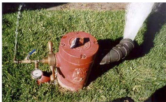
**Figure 2** | Sampling device installed on the fire hydrants.
