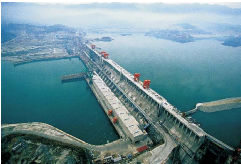
Figure 4. The Three Gorges Dam , being built on the Yangtze River at Yichang, China, is the world's largest hydroelectric project. It symbolizes both China's developmental aspirations and the many problems associated with the country's development trajectory. Although the power it will generate should reduce China's dependence on fossil fuels, it carries a number of economic, environmental, and national security risks.
