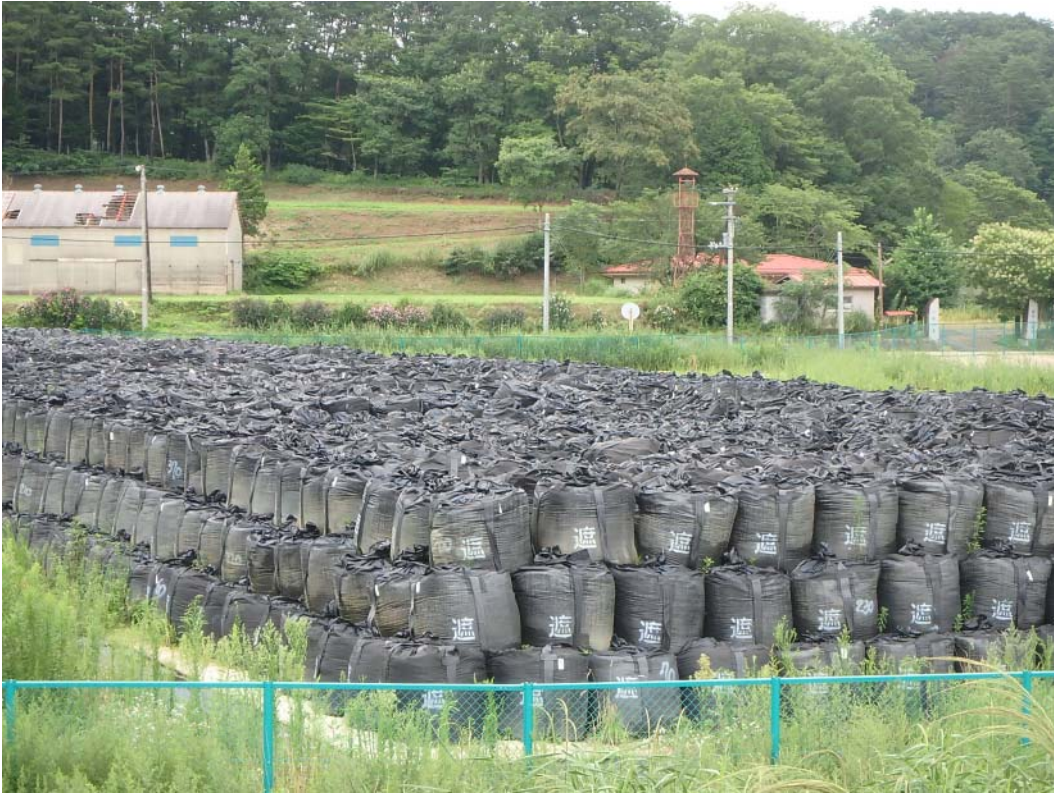
Figure 2. Temporary storage facility in litate for black bags of contaminated soil, 2017. Photograph by the author.
