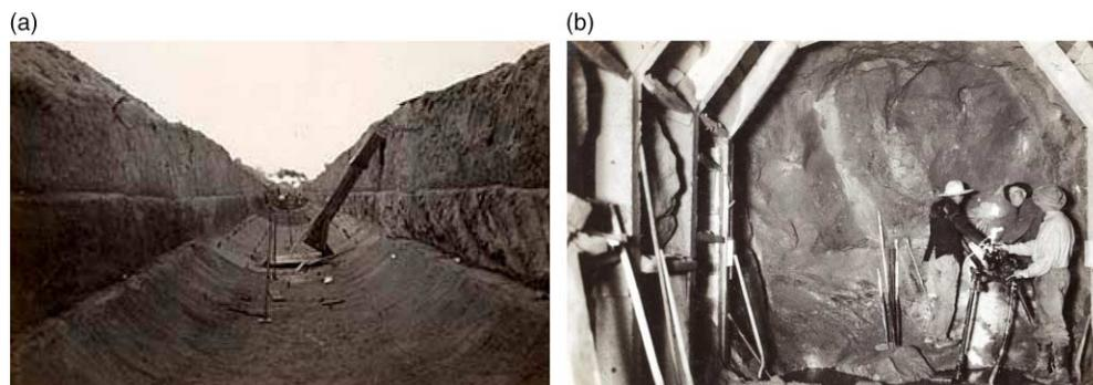
**Figure 3** | First Los Angeles Aqueduct: (a) construction of a box conduit north and east of San Andreas Fault; (b) construction of Elizabeth tunnel passing through the San Andreas Fault. The full colour version of all figures in this paper can be accessed by subscribers online at <http://www.iwaponline.com/jws/toc.htm>
