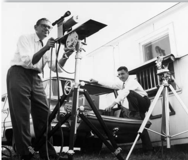
Figure 4. Sending a laser beam 25 miles from Crawford Hill, New Jersey (left) to Murray Hill (right) in 1960. At Crawford Hill, Robert Collins (left) aims a Bell Labs ruby laser at the top of the radar tower in Murray Hill as Willard Boyle prepares to fire it. Atop the tower in Murray Hill, Walter Bond (right) checks the alignment of the photomultiplier detector while Donald Nelson maintains phone contact with Crawford Hill.
