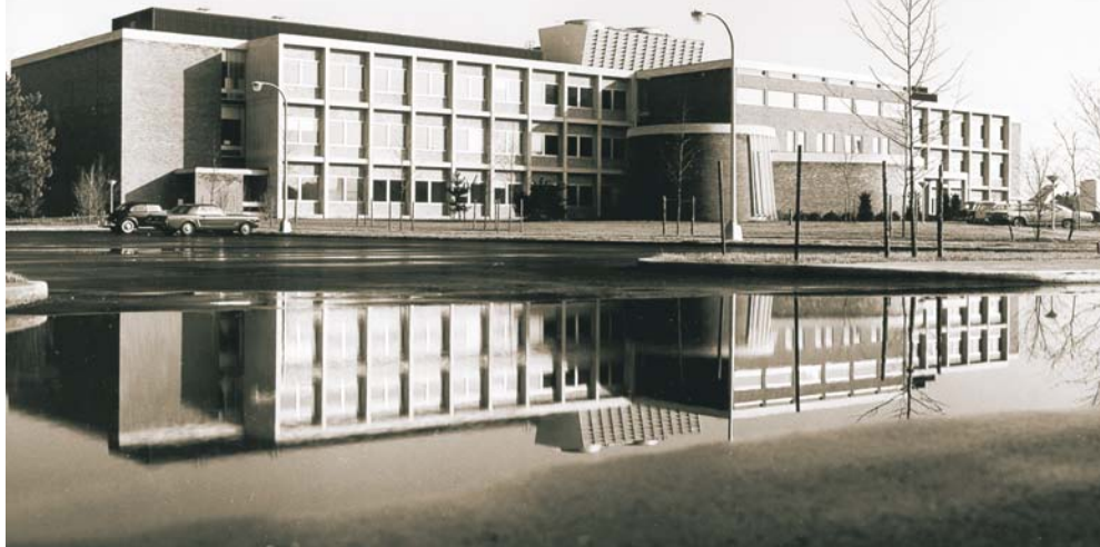
Figure 3. Building 555 , designed by Marcel Breuer, houses chemists at Brookhaven National Laboratory in New York. Nearly 50 years after it opened, the lab is still functionally and technically sound, according to the architectural firm that is currently planning its renovation. (Courtesy of Brookhaven National Laboratory's chemistry department.)
