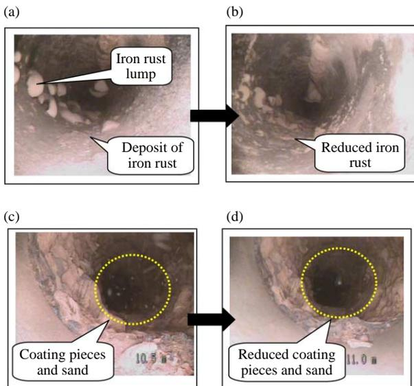
Figure 11 | In-pipe camera view of the inside of the pipes: (a) point A before pipe washing; (b) point A after pipe washing; (c) point C before pipe washing; (d) point C after pipe washing.
