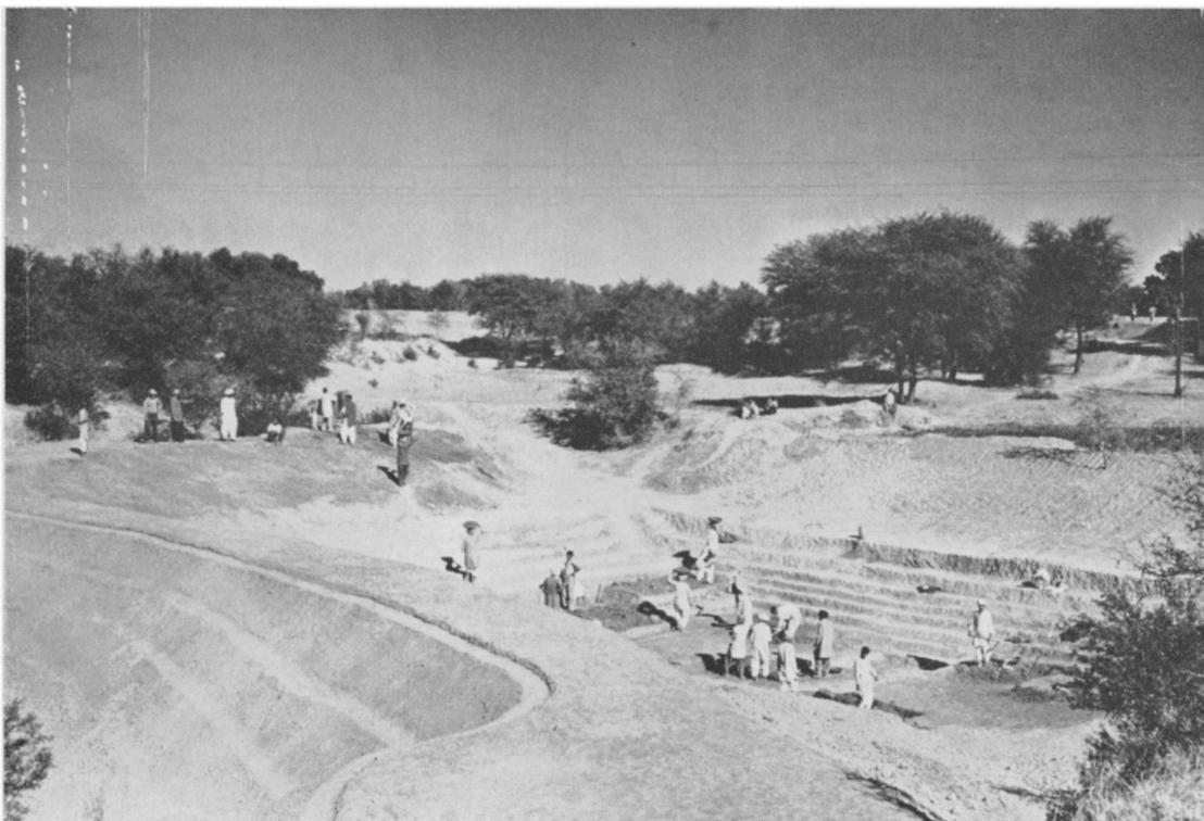
Figure 6. Catchment Basins to conserve water. Most of the rainfall is concentrated during the monsoon summer months, so the excess runoff is collected in such basins, and can be used to irrigate the fields during the dry season.
