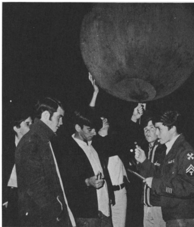
Fig. 6. Students prepare to attach thermometer to weather balloon in order to collect vertical temperature data.
