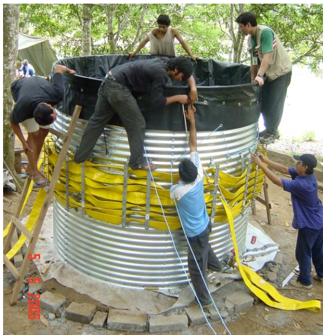
Figure 1 | Construction of the Oxfam Upflow Clarifier in Lamno, Aceh.
