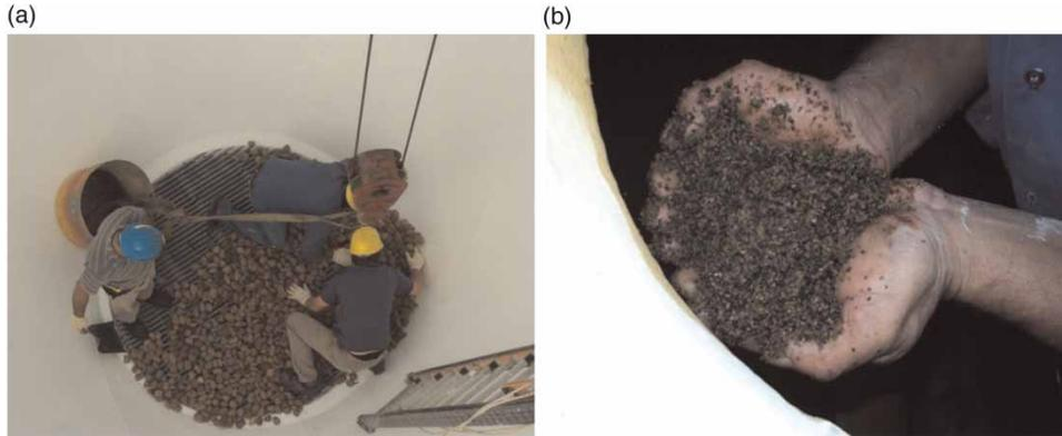
**Figure 9** | (a) Placing gravel in roughing filter (previous circular settler). (b) Filtering material covered with manganese precipitates in rapid filter.
