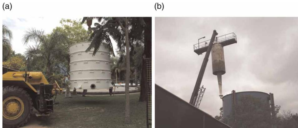
Figure 7 | (a) Incorporation of perforated trays aerator. (b) Retirement of hydro-ejector (incoming system of mixing chemicals at existing circular settler).
