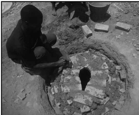
**Photo 5** | Bricks and mud mortar are used to form the pit opening.
