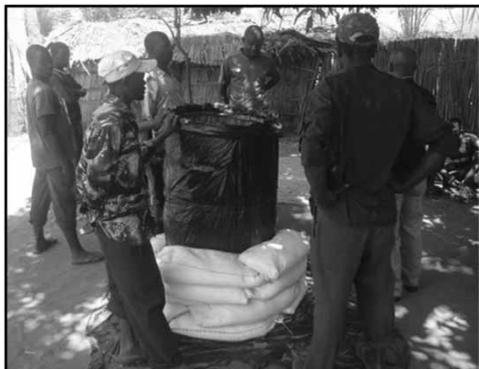
**Photo 7** | Nkhokwe (wooden frame) wrapped in plastic with additional sand-bag reinforcement.
