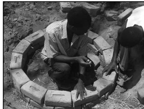
**Photo 6** | Masons use trapezium shaped bricks to form a circular pit lining.
