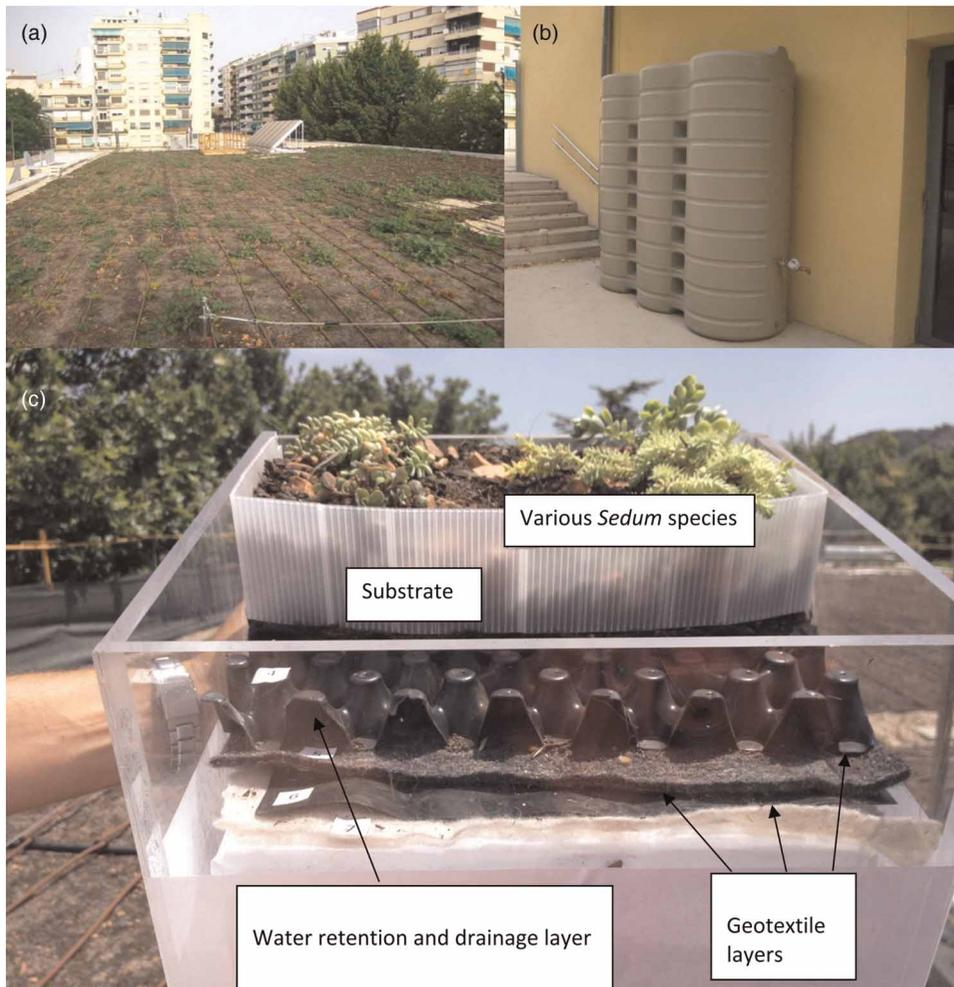
**Figure 5** | Gozalbes Vera Public School SUDS retrofits. (a) Extensive green roof; (b) rainwater tank; (c) structure of the green roof.
