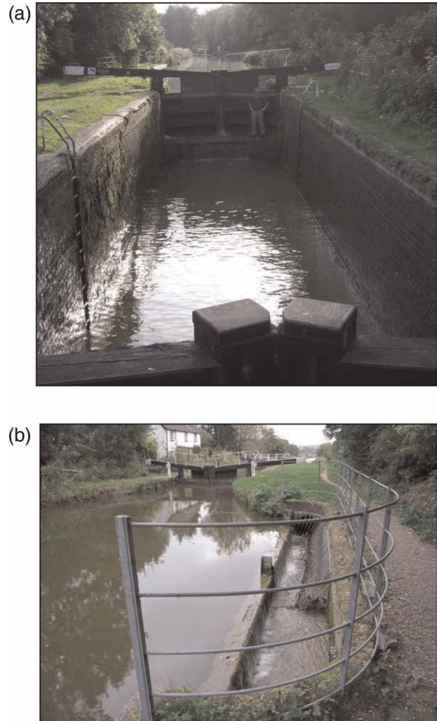
Figure 1 | Photos of a lock and reach on the Kennet and Avon Canal. (a) Interior of a typical lock, (b) part of a reach near the lock gate.
