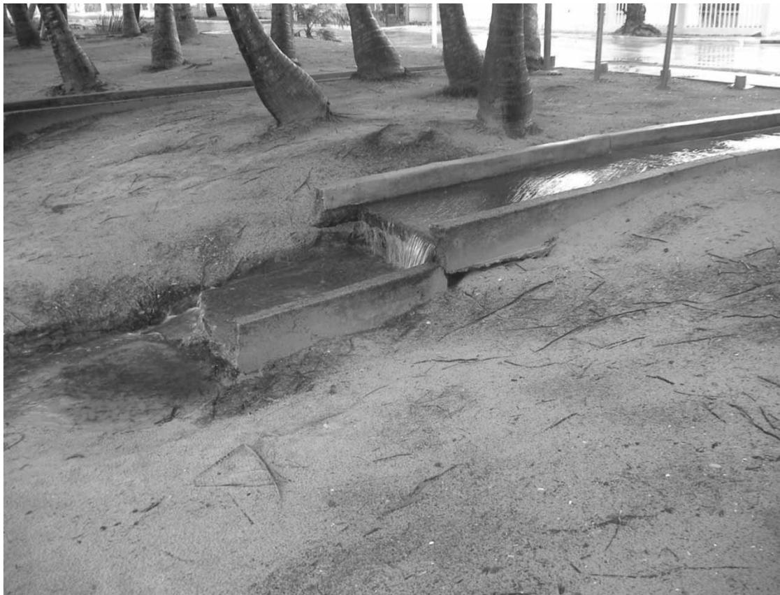
**Figure 2** | Outflow from main culvert draining storm water from residential area into transect 5 of the study area.
