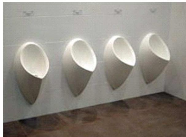
Figure 6 | Improvement of amenity presentation—upgrading a urinal trough to a waterless urinal system.
