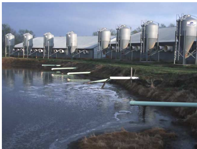
Figure 3 | Swine waste lagoon (Georgia, USA). Photo courtesy of Natural Resources Conservation Service.
