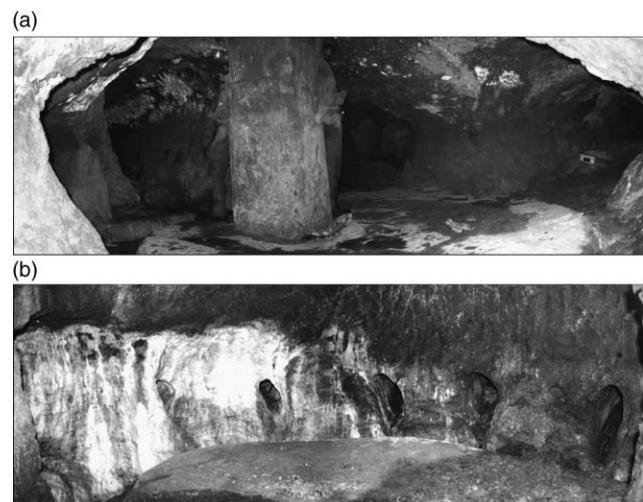
**Figure 6** | (a) Chamber under the shaft number X with the drainage tunnel of last sector of the Springs branch; (b) Particular of the drainage chamber (Capolongo *et al.* 2008).
