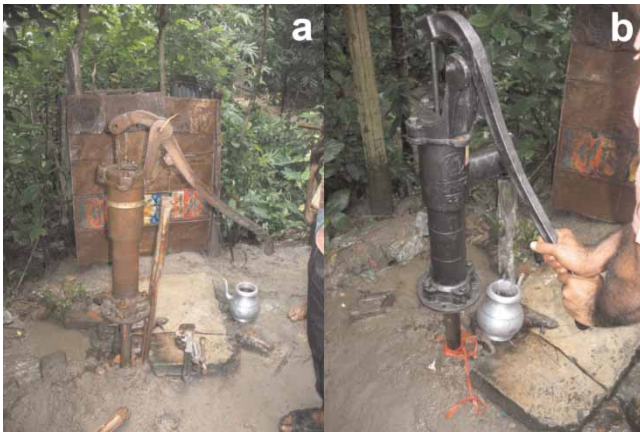
Figure 1 | Tubewell no. 21602 (a) with original hand-pump attached and (b) replaced with a new hand-pump.
