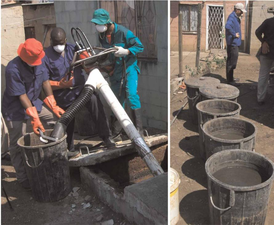
**Figure 5** | Extraction auger being used to empty pit latrine in Durban, South Africa.
