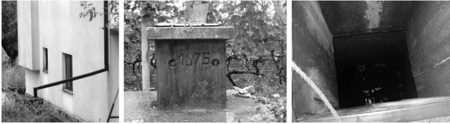
Figure 1 | System for rainwater collecting – ‘čatrnja’.
