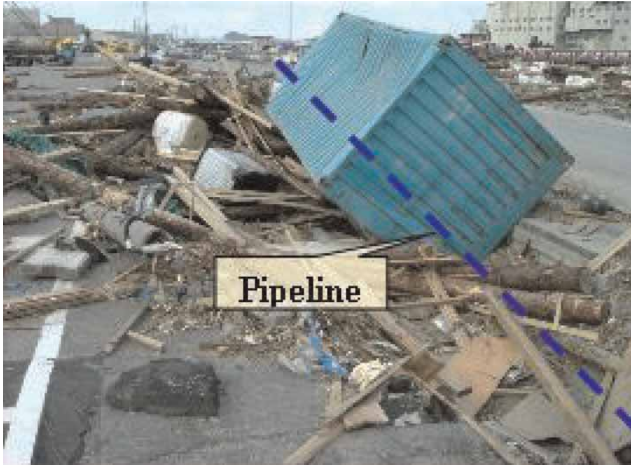
Figure 5 | ERDIP covered by debris.
