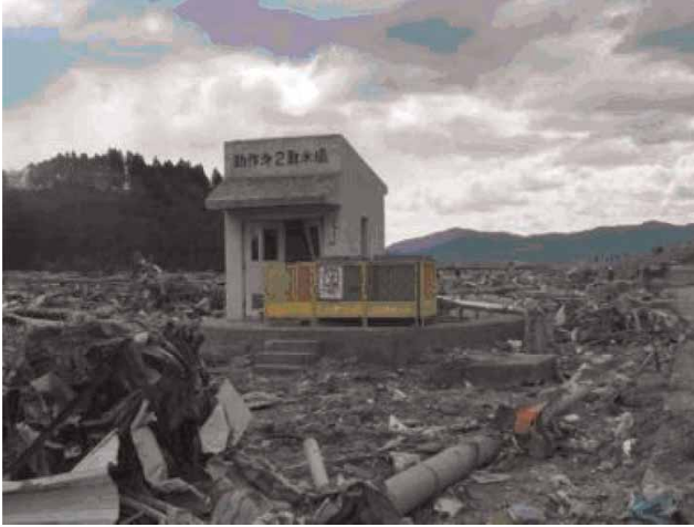
Figure 1 | Inundated intake facilities (Sukedukuri No. 2).
