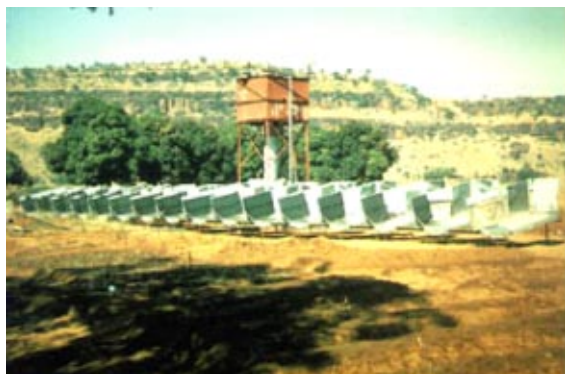
Fig. 3 Solar water pumping plant in Mali with flat collectors and an Ormat ORC turbine
