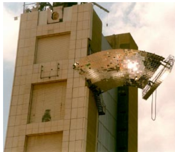
Fig. 9 The Tower Reflector mirror prototype installed on the Solar Tower at the Weizmann Institute
