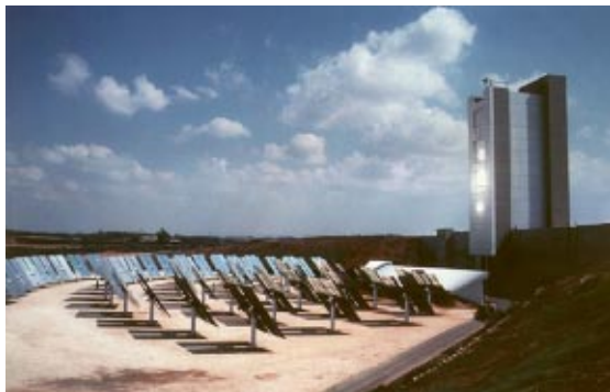
Fig. 7 The solar tower and heliostat field at the Weizmann Institute of Science
