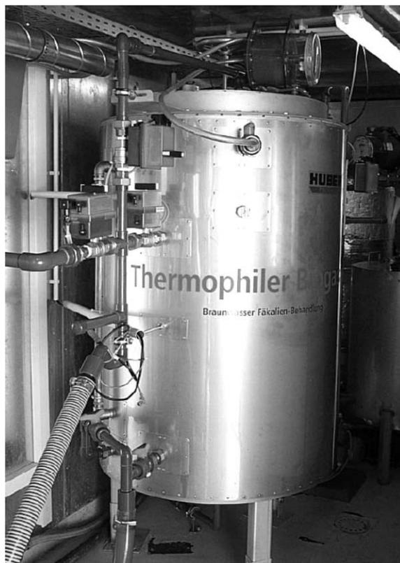
**Figure 1** Thermophilic anaerobic bioreactor
