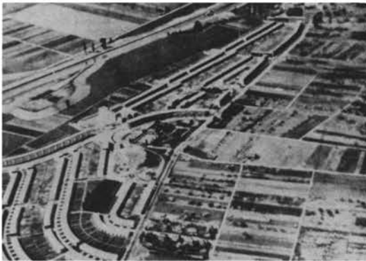
3 Housing estates on the suburban fringe: Römerstadt in Frankfurt by Ernst May, 1925–1930.
