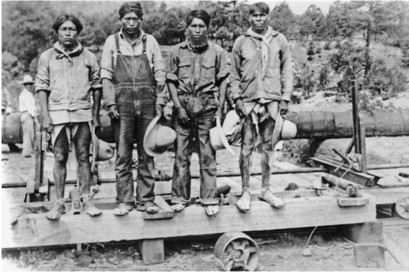
Figure 3.3. Directive Council of the Cusárare ejido and cooperative during construction of a sawmill in the village of Yahuir, ca. 1948. Archivo General de la Nación, SARH/PF, caja 1575, exp. 28, leg. 3.
