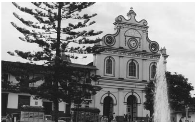
Figure 4. Church of San Sebastián, on the Upper Plaza, 1994
