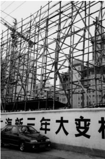
A residential area in central Shanghai in the process of being demolished. (Photo by Zhang Zhen)
