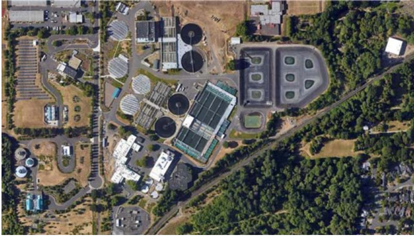
Figure 6.1 Durham advanced wastewater treatment facility.
