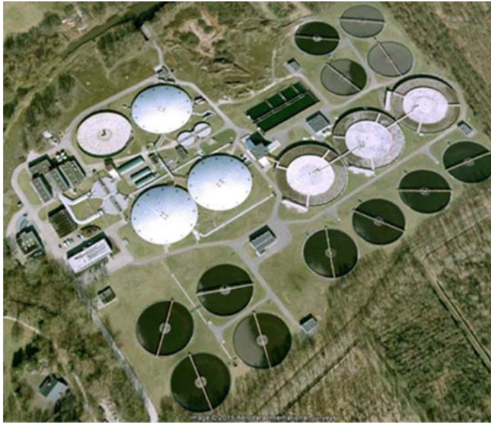
Figure 6.6 Aerial view of the Eindhoven WWPT.
