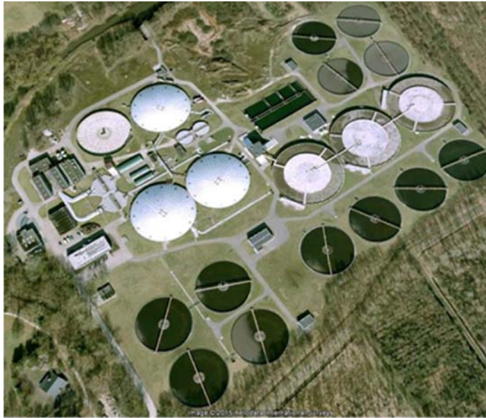
Figure 6.6 Aerial view of the Eindhoven WWPT.
