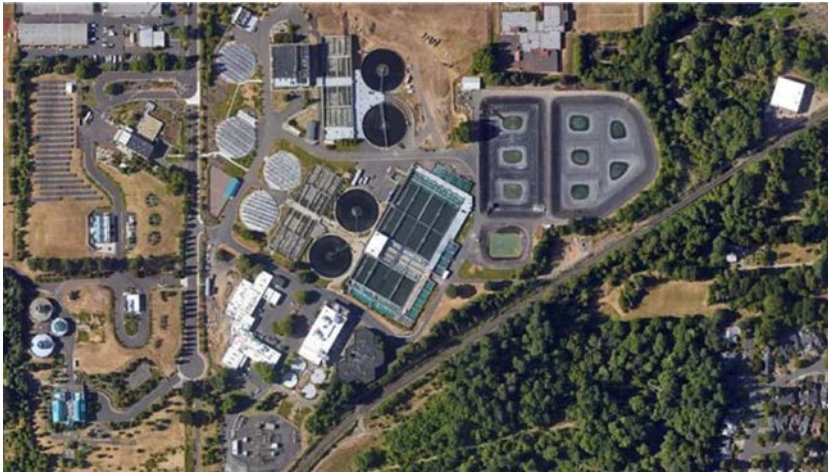
Figure 6.1 Durham advanced wastewater treatment facility.
