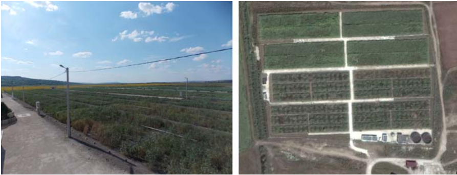
Figure 6.9 Case study 7 – Orhei Wastewater Treatment Plant (Moldova).
