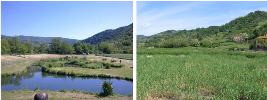
Figure 6.8 Case study 6 – Dicomano Wastewater Treatment Plant (Italy).
