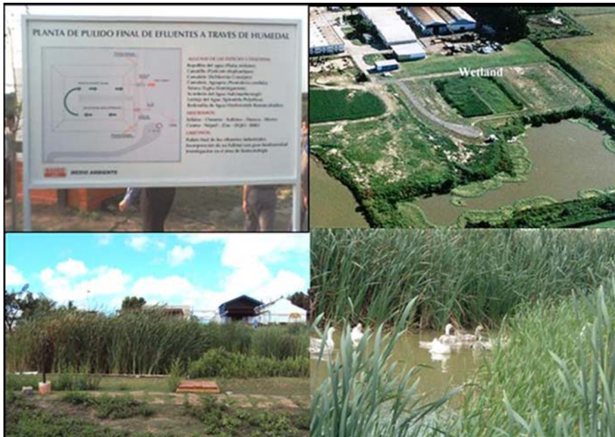
Figure 6.12 Case study 10 – Bahco treatment wetland for effluent final polishing (Argentina).
