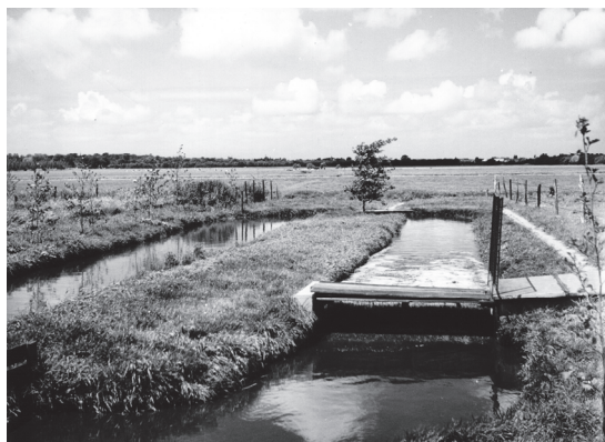
Figure 1.2 The first (pilot) application of the Pasveer ditch system (at Voorschoten, The Netherlands in 1954). The plant capacity was 400 P.E. and 40 m 3 /h at dry weather flow (photo: Van Lohuizen, 2006).
