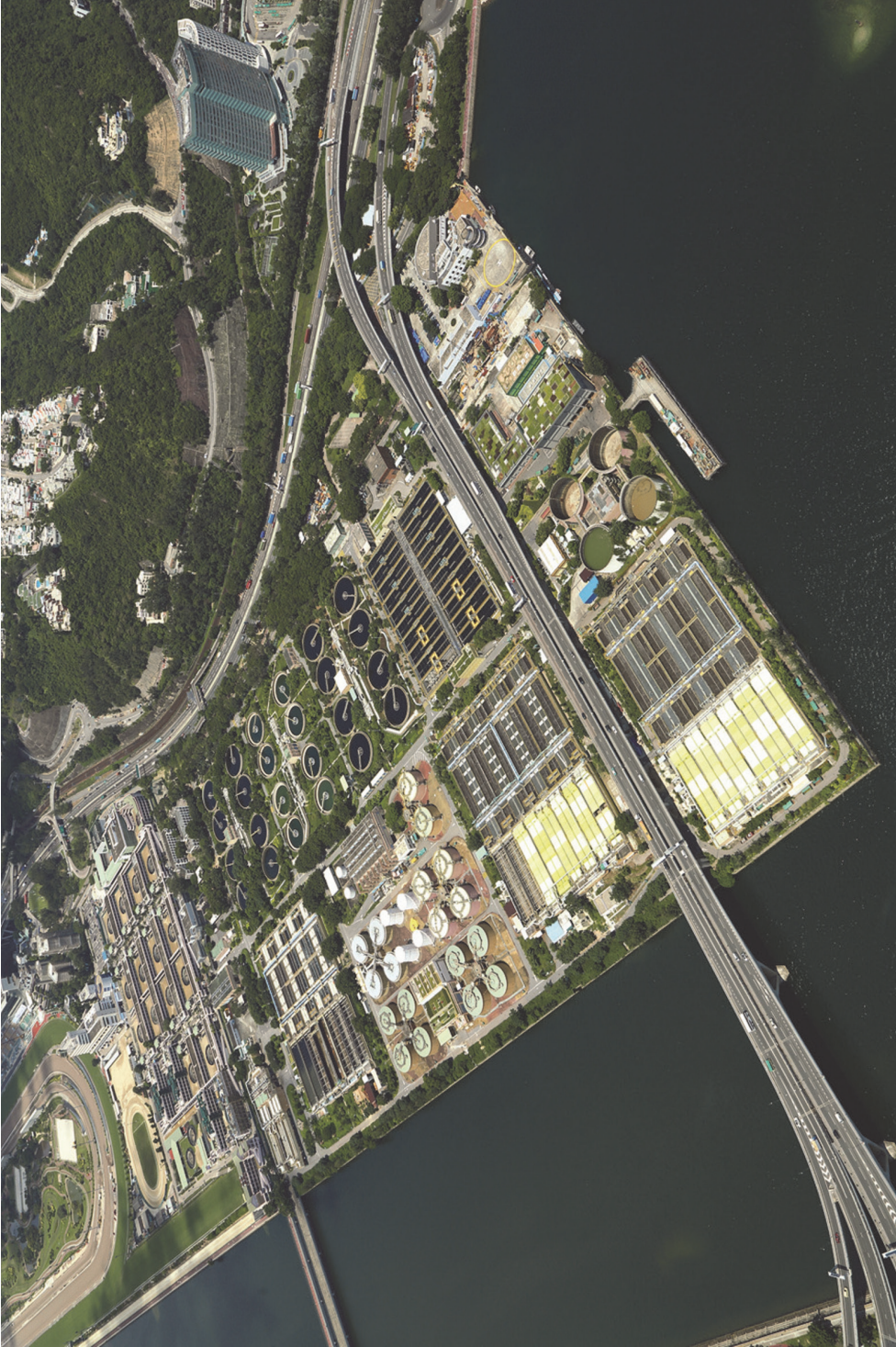
Figure 1.3 An example of a state-of-the-art wastewater treatment plant: Sha Tin Sewage Treatment Works in Hong Kong (photo: Drainage Services Department, HK).
