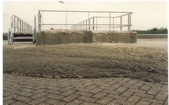
Figure 10.11 Extreme manifestation of sludge bulking (photos: Eikelboom, 2006).
