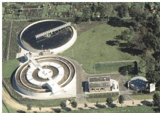
Figure 10.1 A modern biological nutrient removal plant in The Netherlands (BCFS® process) showing the importance of sludge separation on the total process layout. The settling tank design was based on a sludge volume index (SVI) of 120 ml/g (photo: Van Loosdrecht et al. , 1998).
