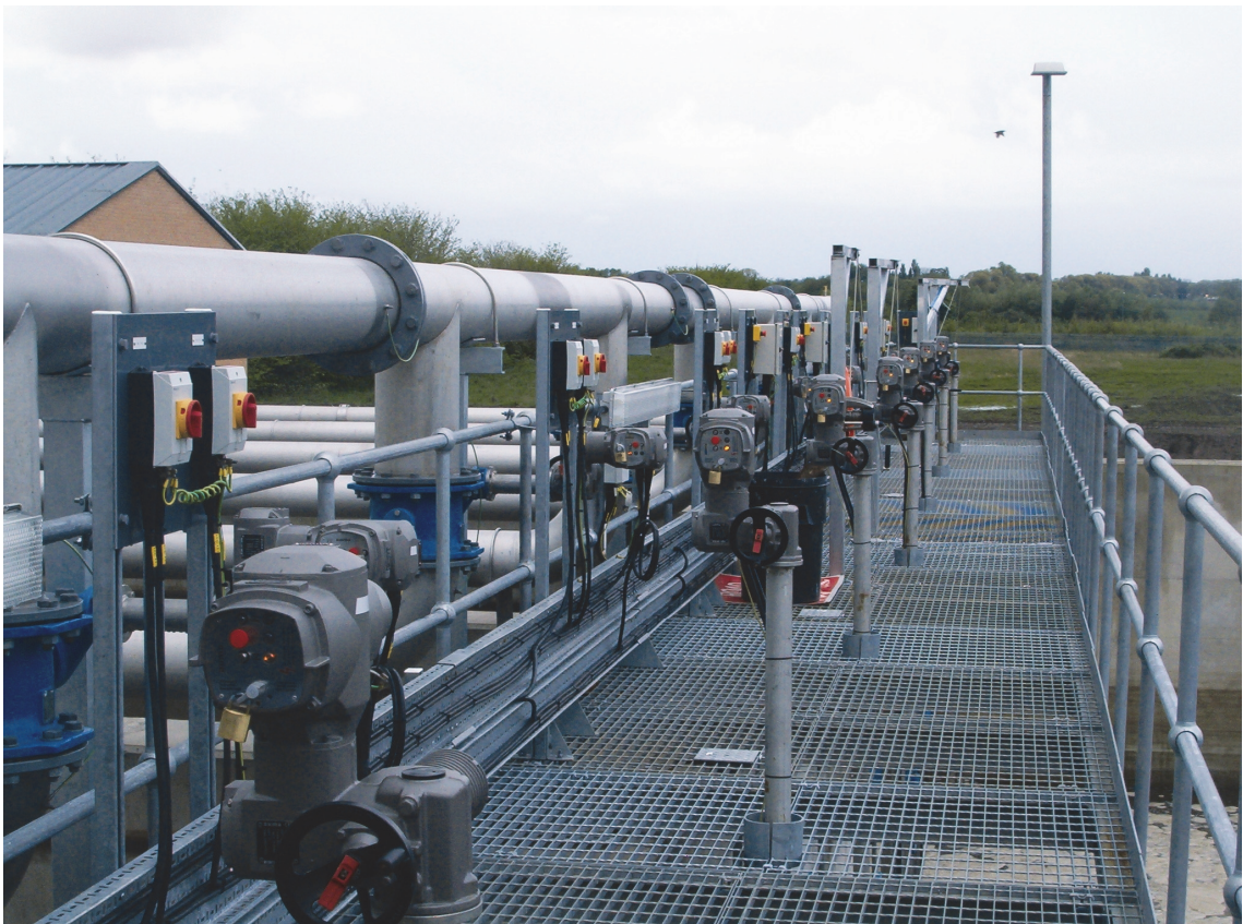
Figure 15.16 Detail of measuring and control system of activated sludge aeration tank (photo: D. Brdjanovic).
