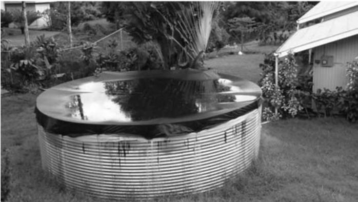
**Figure 4.8** Permeable ground cover cloth commonly used as tank cover. (Source: Authors).
