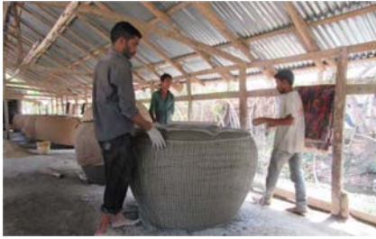
Figure 7.7 Reinforcement with wire net. (Source: Author's own).
