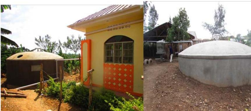
**Figure 9.1** 50 m<sup>3</sup> ferrocement tanks. (Source: Kikundwa Anne).
