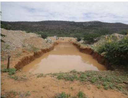
Figure 16.5 A four-meter deep trench-like rock cistern stores water for goats. (Source: Author).
