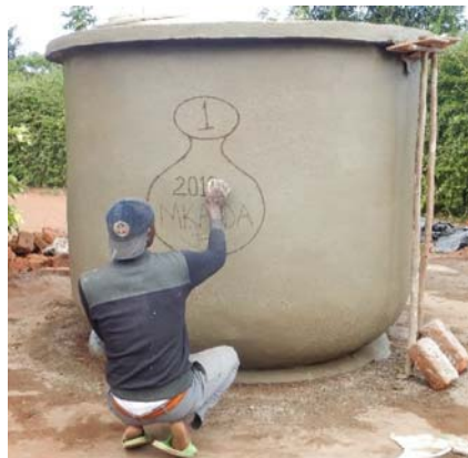
Figure 18.6 Finishing the outside. (Source: Author's own).
