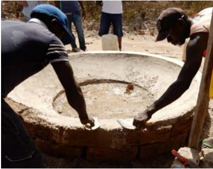
Figure 18.3 Preparing the hollow part of the mould. (Source: Author's own).
