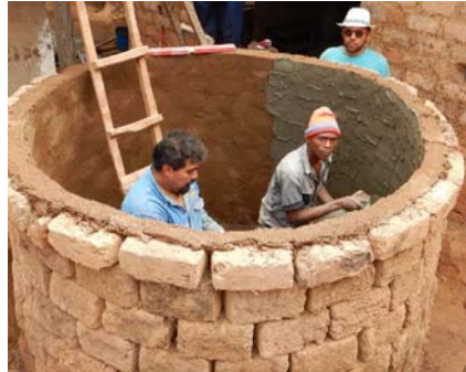
Figure 18.4 Plastering the inside of the mould. (Source: Author's own).
