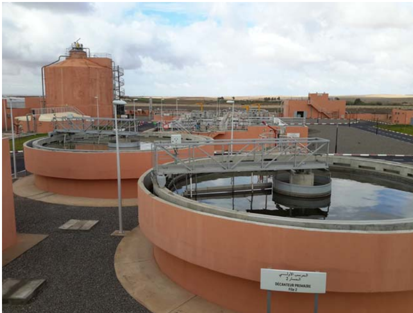
Figure 6.8 Benguerir's wastewater treatment plant. (Credit. OCP).
