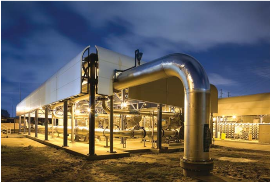
Figure 23.1 West Basin's Edward C. Little Water Recycling Facility (El Segundo, CA) treats 150 ML/d (40 mgd) of secondary effluent to non-potable and potable standards for municipal and industrial reuse. (Credit: West Basin Municipal Water District)
