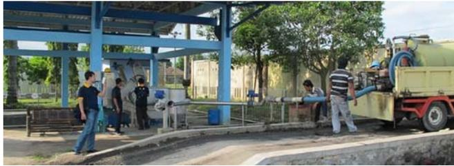
**Figure 1.4** Septage treatment facility is an important component of scheduled desludging schemes. Their capacity often becomes the limiting factor that determines the coverage of septage desludging scheme in the early years.
