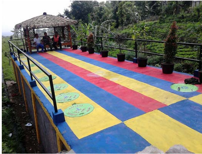
Figure 6.2 Community-based wastewater system uses a treatment unit that also require periodic sludge removal services. If agreed, they can also be the target of the scheduled desludging service.
