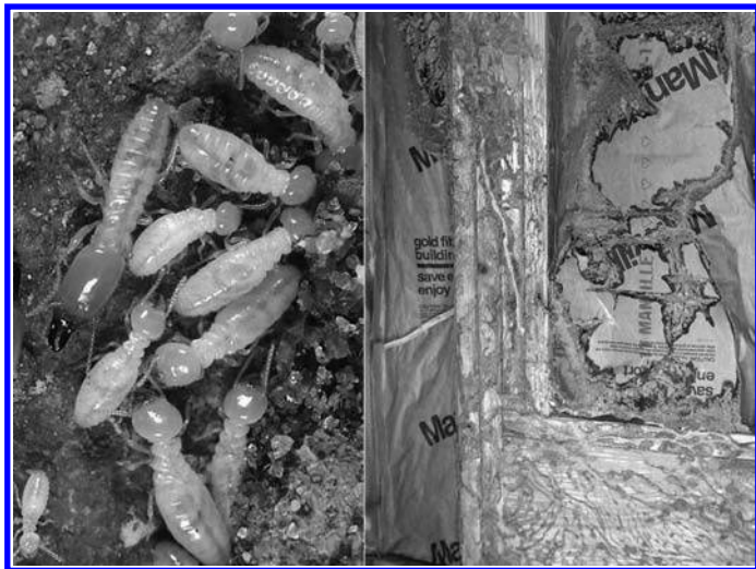
Figure 1. (Left) Reticulitermes , North America's common subterranean termite; the individual with the larger, darker head is a soldier; both soldiers and workers are blind. (Right) Hidden termites have eaten away the wallboard shown exposed here.
