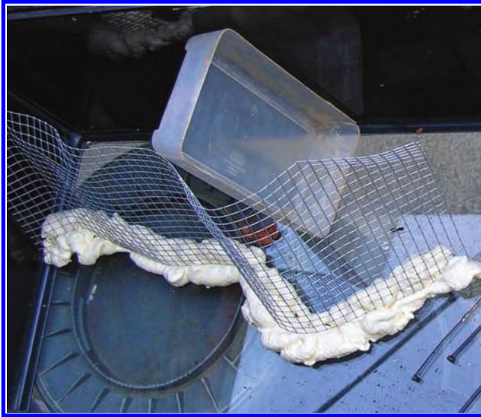
Figure 1. Hardware cloth being shaped to create a back wall. The same material can be shaped and attached to make planters.
